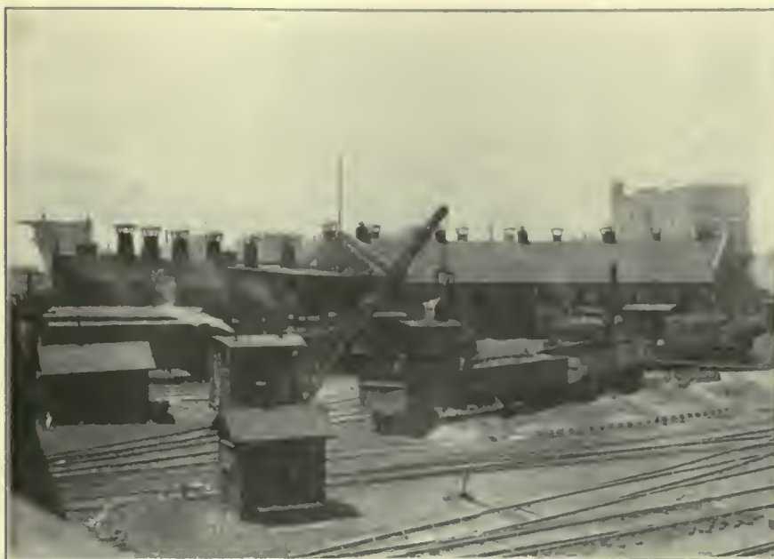
FIG. 663. FACILITIES TO BE ABANDONED. Locomotive engine house of the Chicago, Burlington & Quincy Railroad, near 12th and Canal streets. This house has 15 stalls, each 60 feet long, and in the event of electrification, would be a total loss, since the materials are not suitable for use in new construction.
